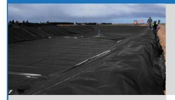
Aquamark® is a high quality Polypropylene based polyfabric designed for lining ponds and dams. Aquamark® consists of the PP base scrim with a highly flexible, UV stabilised PP coating; supplied in bulk rolls.
