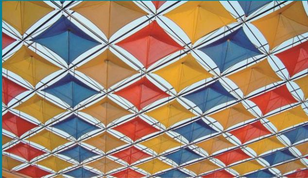
Commercial 95® is a high quality knitted shade fabric designed for tension structures, awnings and shade covers specifically for commercial architectural applications; supplied in bulk rolls.
