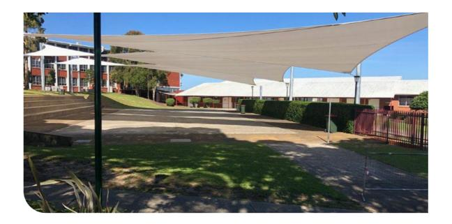
Bleachers built at the edge of the space were popular for both students and teachers alike, and covering them would mean the sails would need a huge 33 metre span. This in turn necessitated larger columns to support the sails' weight, with a diameter of 323mm.
